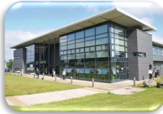
IBM campus Dublin, Ireland
